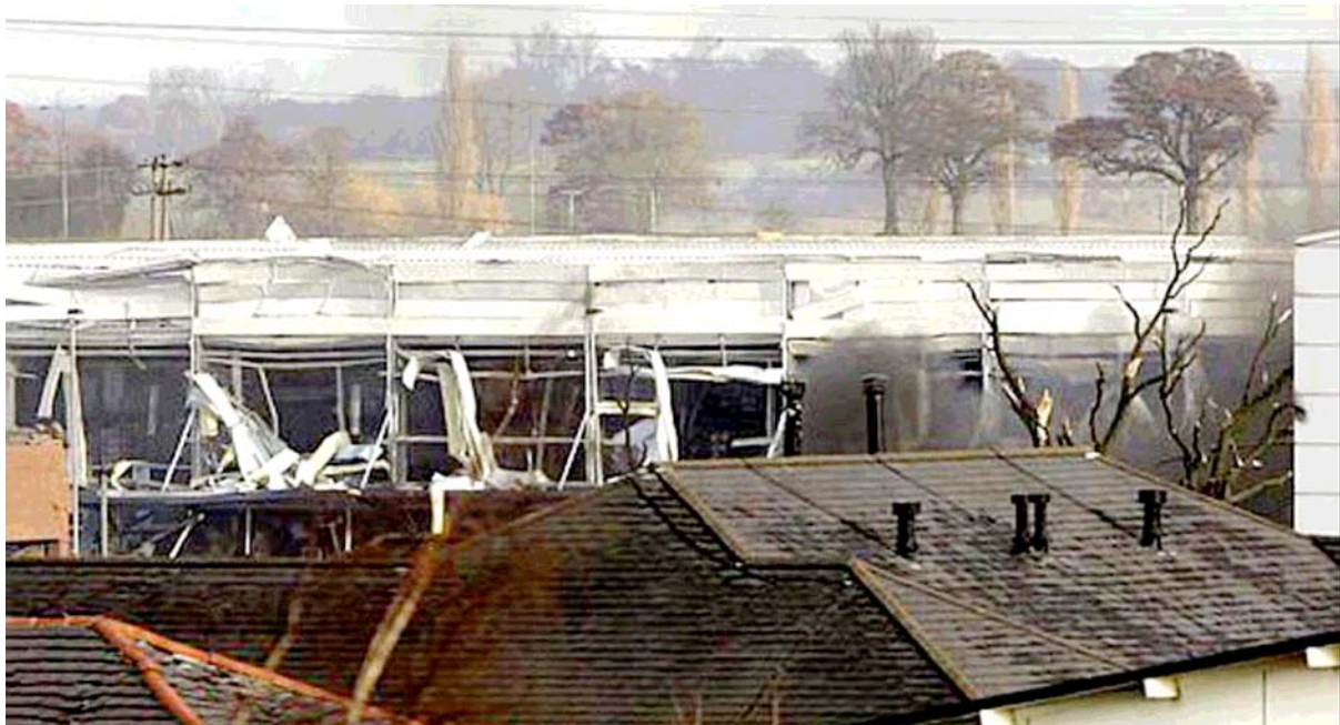
Metal façade destroyed along the whole length of Hall (5)
