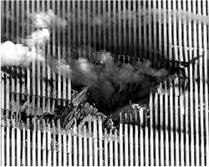
Figure 5: Impact damage to the north face of WTC 1 [3]
